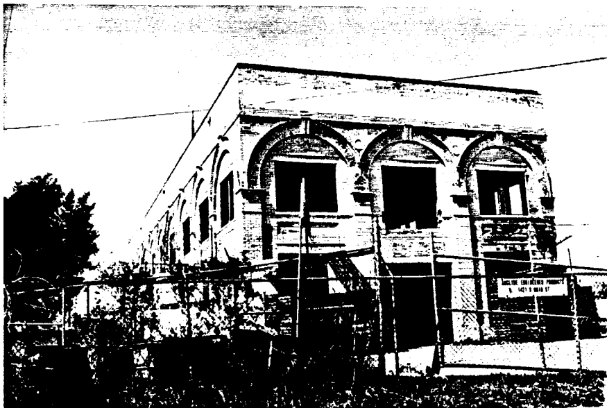
Figure 72: Photograph of a Warehouse
