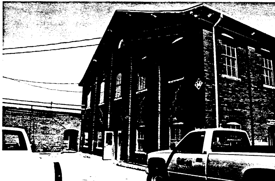
Figure 34: Photograph of Filtration Building at Moore's Bridges Water Treatment Plant
