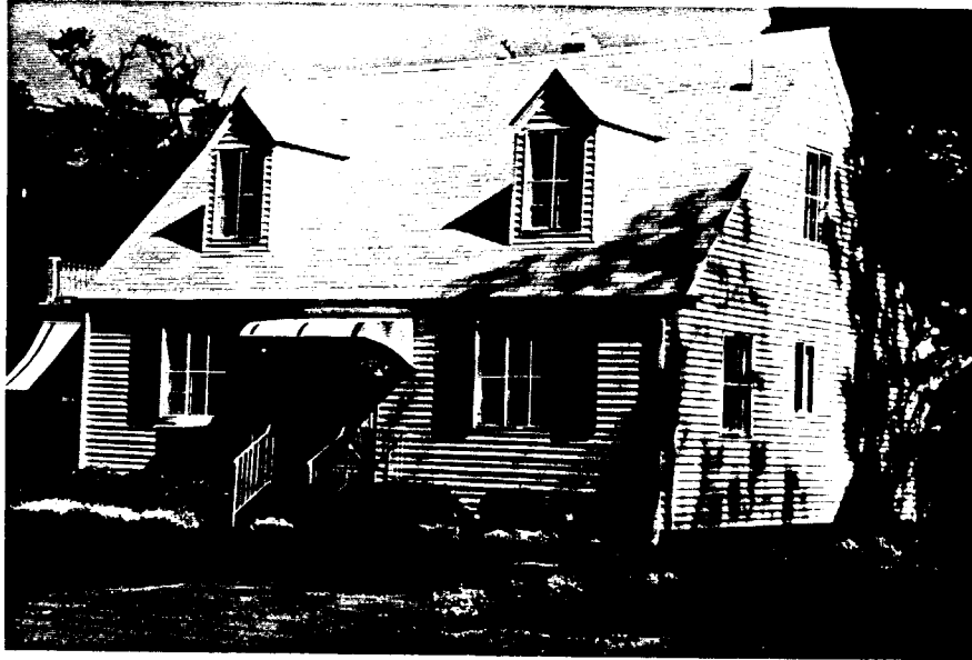
Figure 28: Photograph of House, 402 Ashlawn Drive
