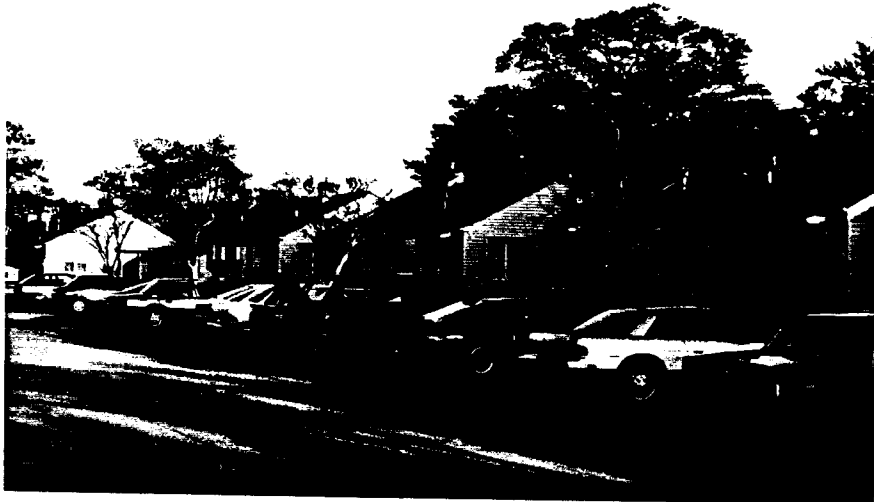
Figure 29: Photograph Merrimac Landing of Apartments
