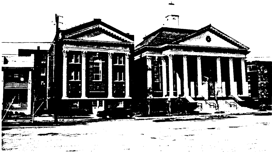
Figure 48: Photograph of Park Place Church
