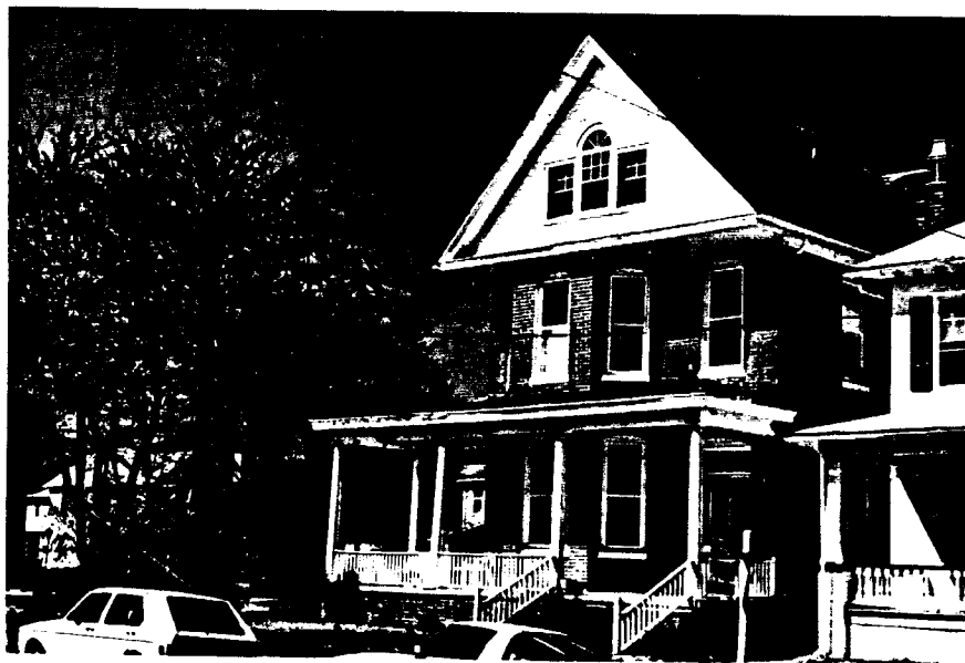
Figure 16: Photograph of Dillard House
