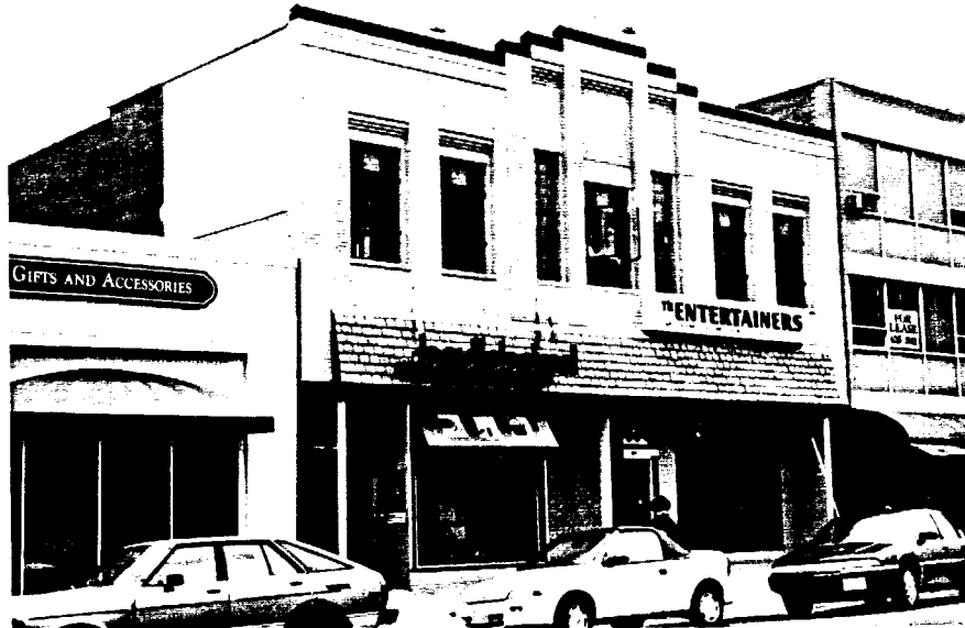
Figure 73: Photograph of 1611 Colley Avenue Building
