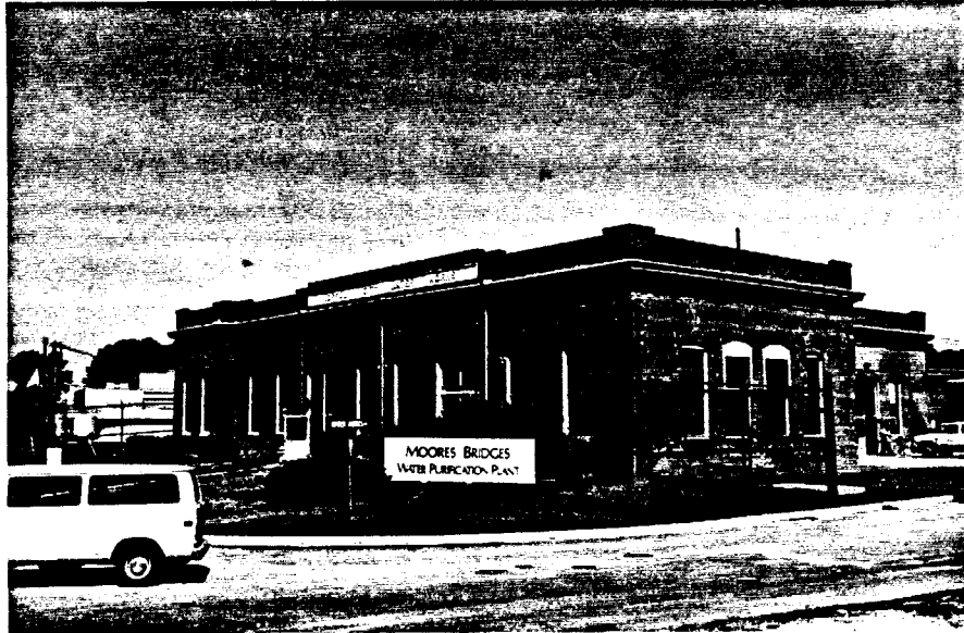
Figure 33: Photograph of Pumping Station at Moore's Bridges Water Treatment Plant
