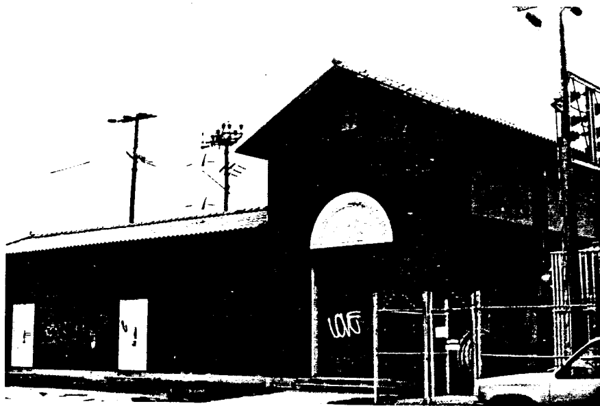
Figure 78: Photograph of McLaughlin Substation
